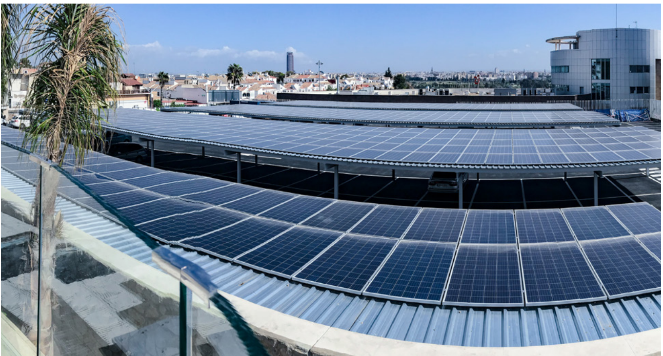
Photovoltaikanlage Gran Casino in Sevilla
